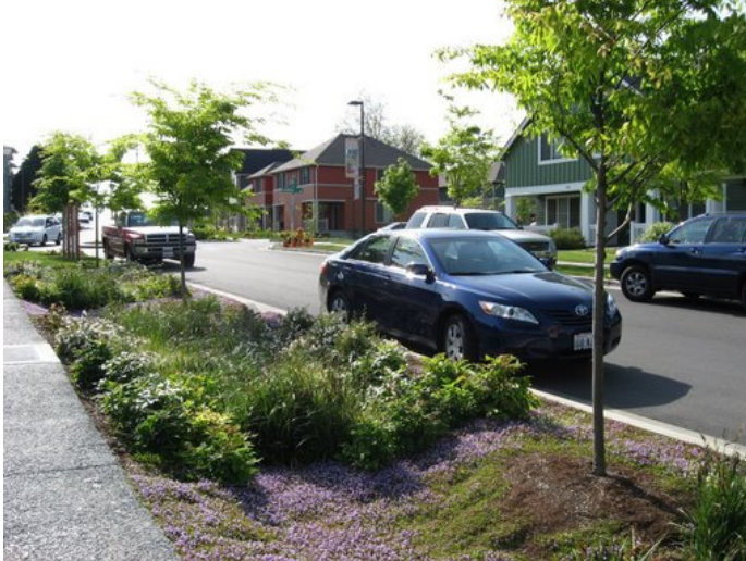
Figure 1. The street-side swale and adjacent porous concrete sidewalk are located in the High Point neighborhood of Seattle, WA (Source: Abby Hall, US EPA).
